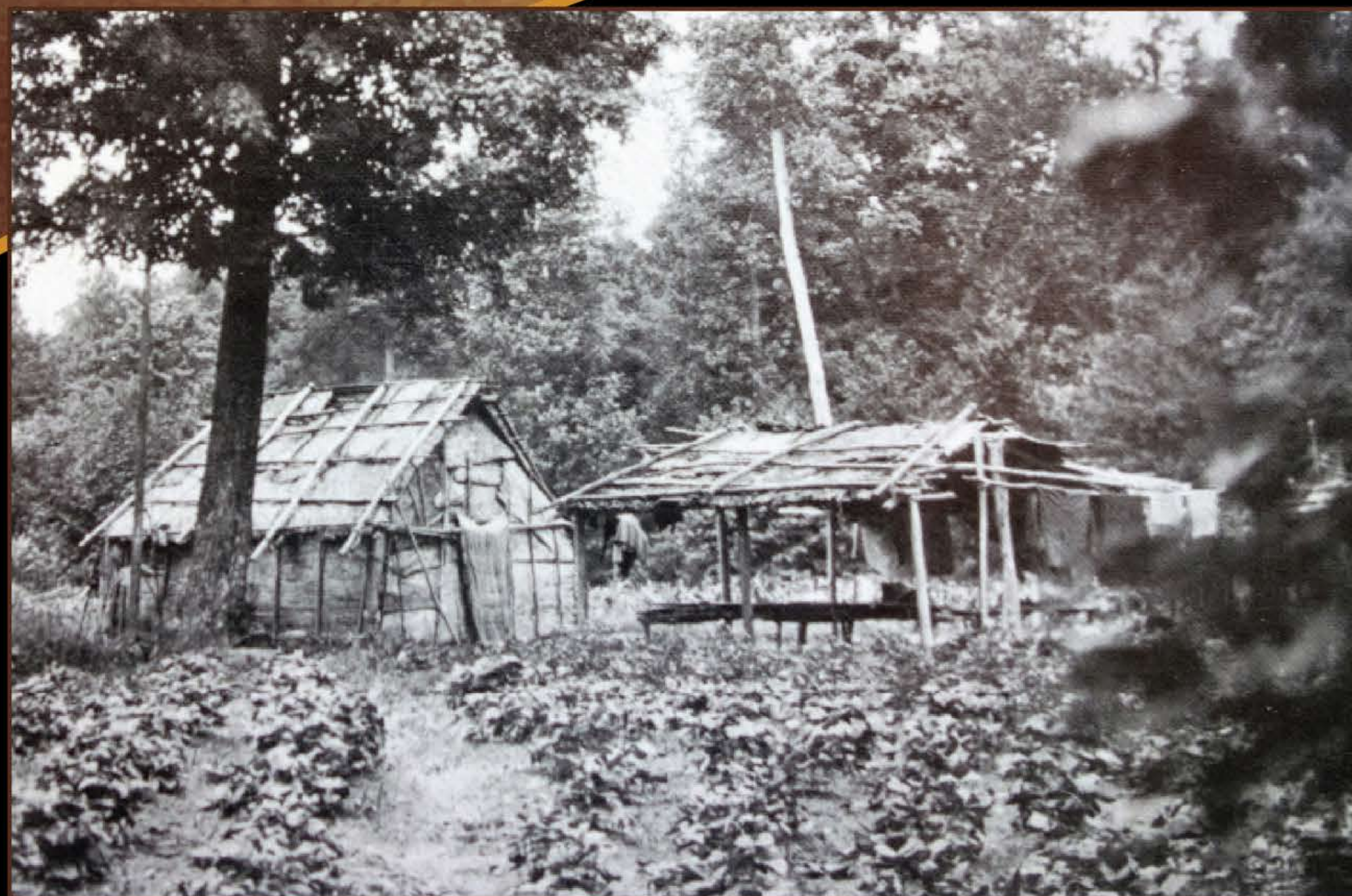
▲ Potawatomi summer houses were much larger than winter homes. Summer houses were built with a rectangular frame of saplings, covered with elm bark, and had an arched roof or could be a large domed shaped wigwam. From Native American Architecture by Peter Nabokov and Robert Easton.
