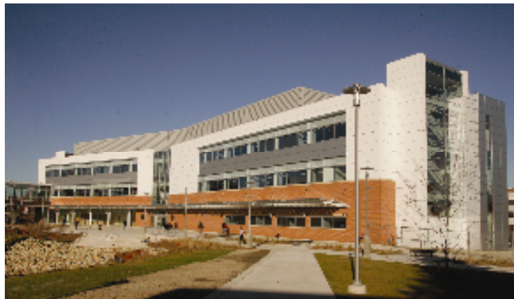
$28.5 million chemistry building (opened 2007)
